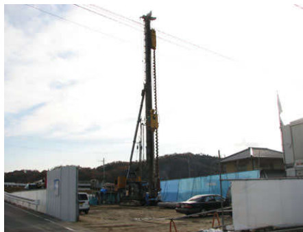
The construction of the new HEC
